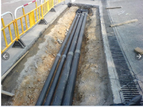
(3) Laying of Spare PVC Duck
