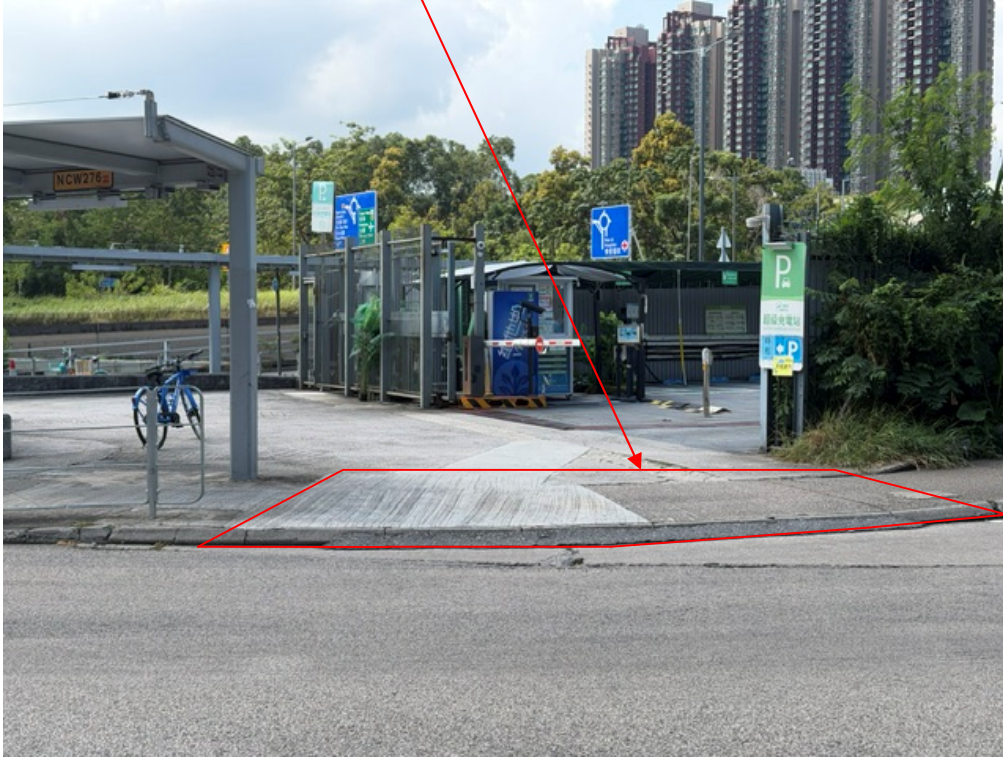
Photos of Existing Condition of Proposed Run in/out
